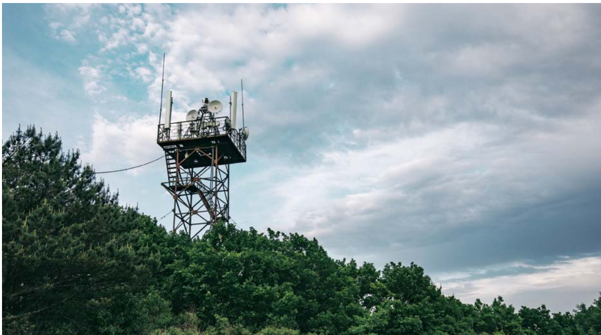
An LTE base station in the Northeastern China Tiger and Leopard National Park that reuses existing fire towers
